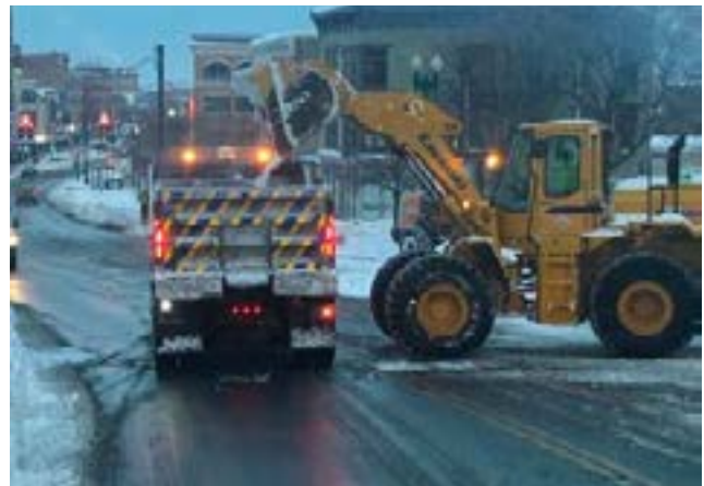
DOT truck being loaded by a loader.
